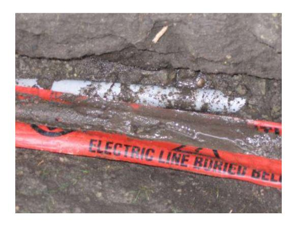
This is what the marking tape looks like. The wiring is on the bottom of the trench, then the trench is filled  $\frac{1}{2}$  way to the top then the marking tape is installed and the backfill is completed.
