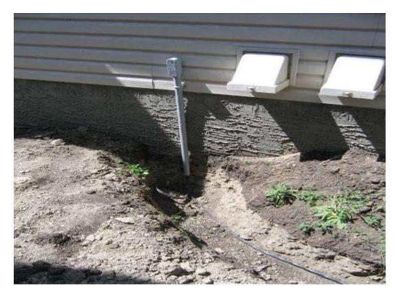
This is installation method #2 - NMWU cable direct buried - one continuous cable running from the house panel to a junction box or panel installed in the garage.
