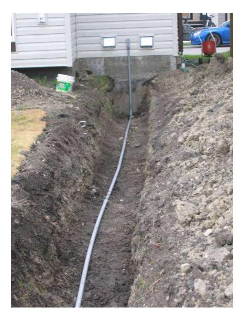
This is installation method #1 - NMWU cable in Rigid PVC Conduit - one continuous cable running from the panelboard in the house to a junction box or panel installed in the garage. The cable is protected by PVC conduit on all exterior surfaces and for the entire underground section. Must be buried a minimum 18".
