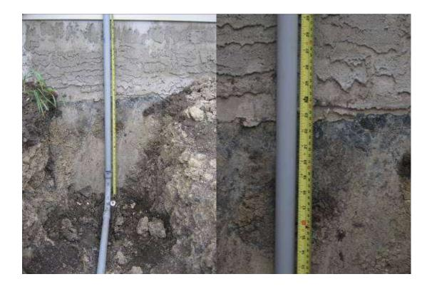
If the trench needs to be back-filled prior to the inspection day, you must present clear evidence of the wiring method and the depth of the trench. Photos taken with a tape measure in the trench showing depth are acceptable or you can leave one end of the trench open (at either the house or garage end). These 2 photos above along with a photo showing the long view of the trench (such as in the previous photo) are the type of photographic evidence that is required.
