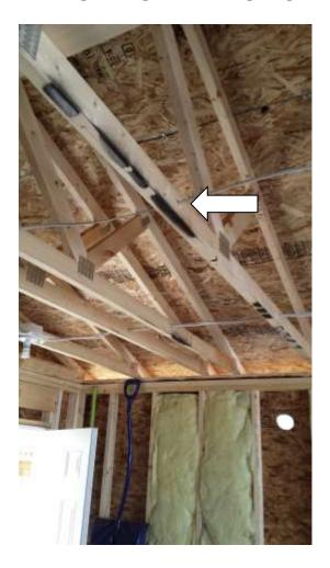
This is a major mistake – NEVER DRILL THROUGH THE TRUSSES. Wire can be laid on top of the trusses then stapled within 300mm (12") of the light box or door opener receptacle box. If trusses are drilled (or otherwise damaged) the truss manufacturer or a structural engineer must provide a repair procedure.
