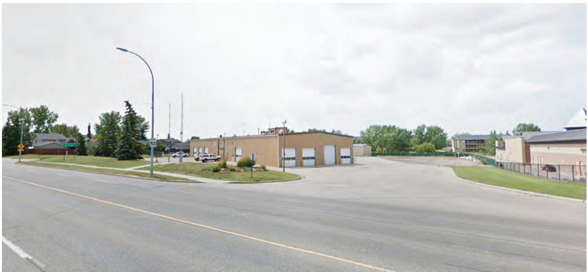
▲ Street view looking south-west at the project site
