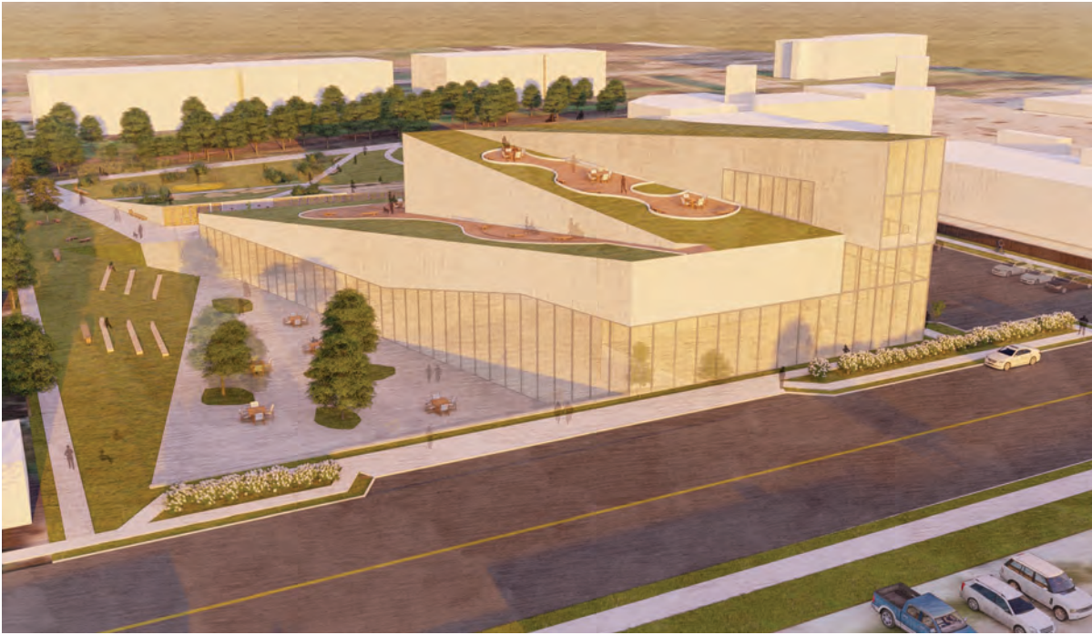
▲ Aerial perspective looking west above the public plaza, building street frontage, and landscaped roofs
